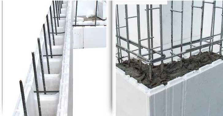
Fig. 2. Construction process of ICF wall structure (ARFA Construction Website)
