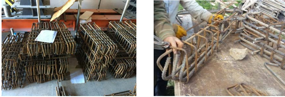
Figure 3. Production of balanced reinforced cantilever beam
