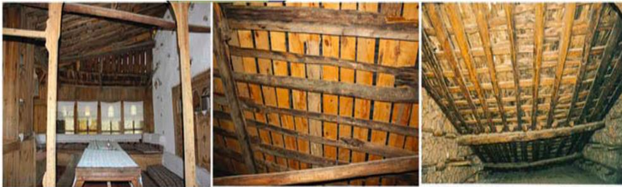
Figure 9: Typical Roof Types In the Village(Sağiroğlu, 2017)
